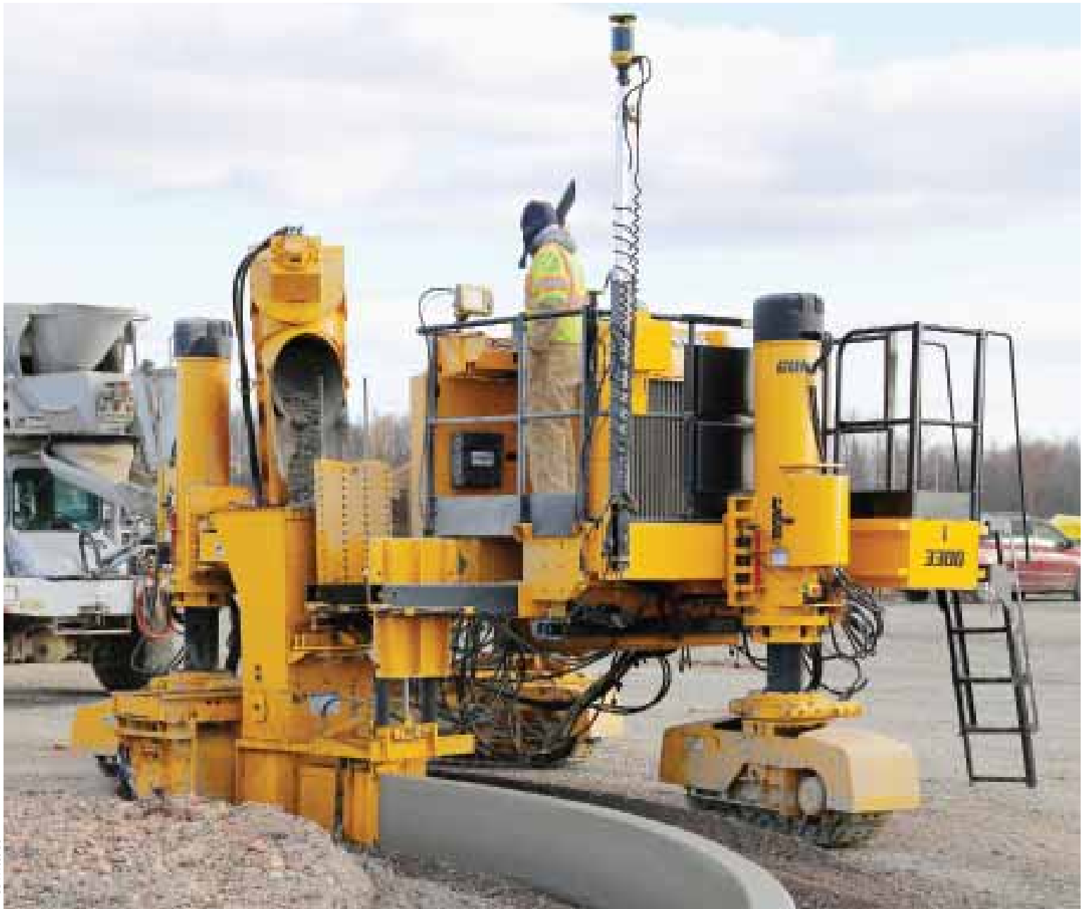
This GOMACO 3300 is slipforming an 18 inch (457 mm) stand-up curb using 3D machine guidance.
