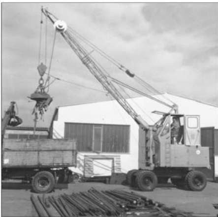
1962: Rope-driven S833 with elevated cab
