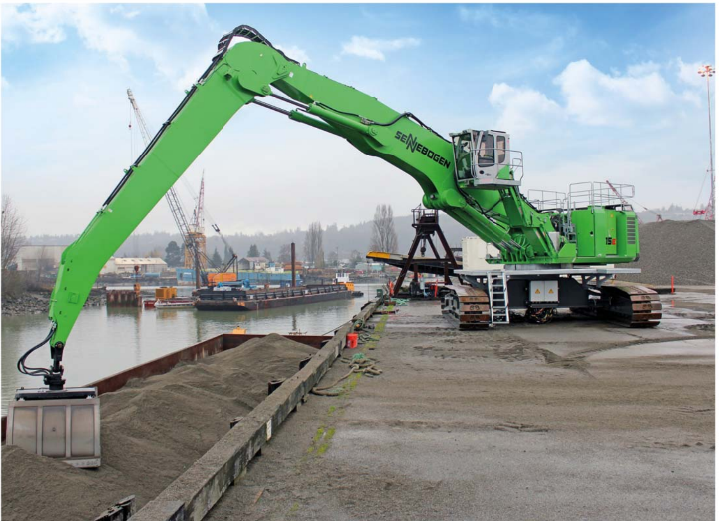
Port handling using a double-shell grab, USA
