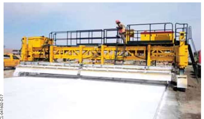
The GOMACO T/C-5600 texture/cure machine has the structural integrity to apply texture and cure up to 56 feet (17.1 m) wide.
