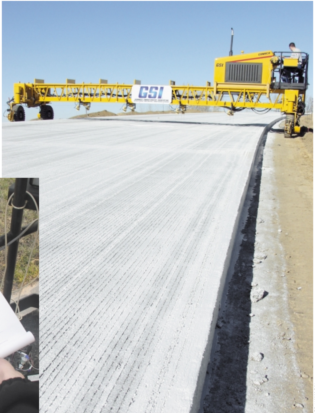
The GSI measures pavement smoothness behind the texture/cure machine on a project near Onawa, Iowa.
